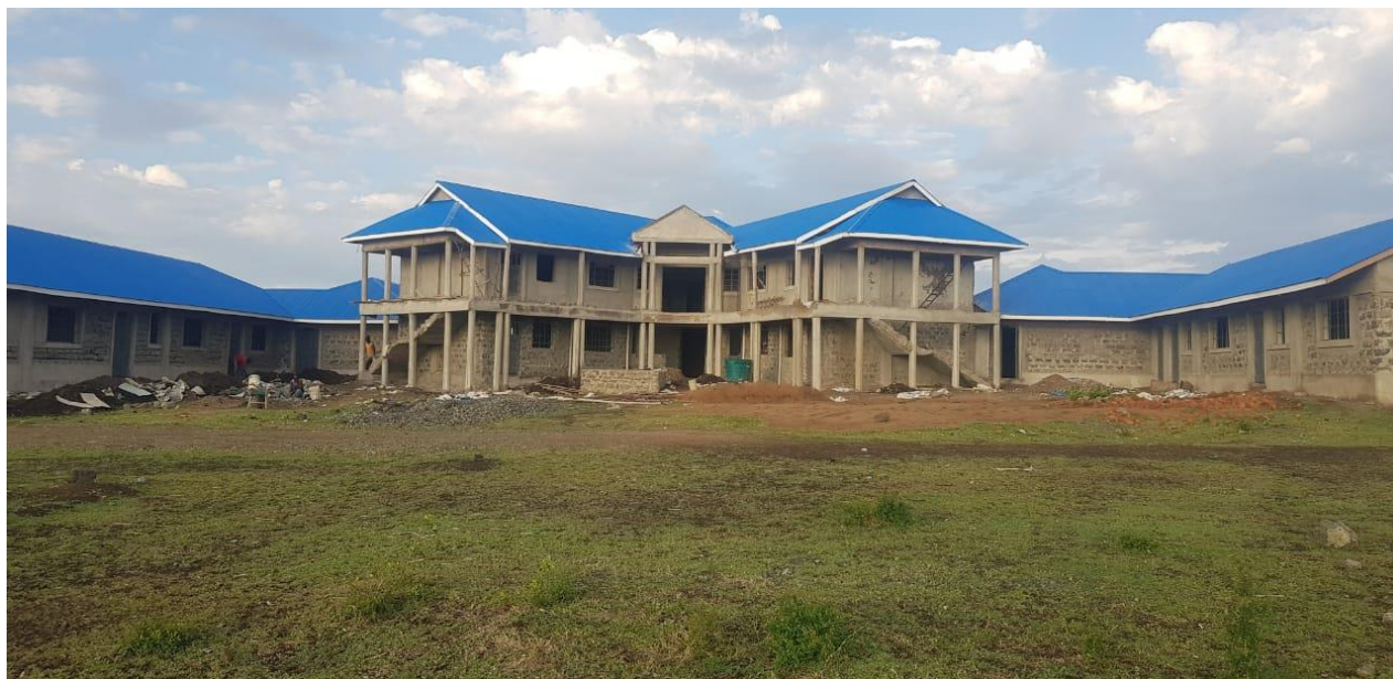
De Madaras school in Okayo village in aanbouw
